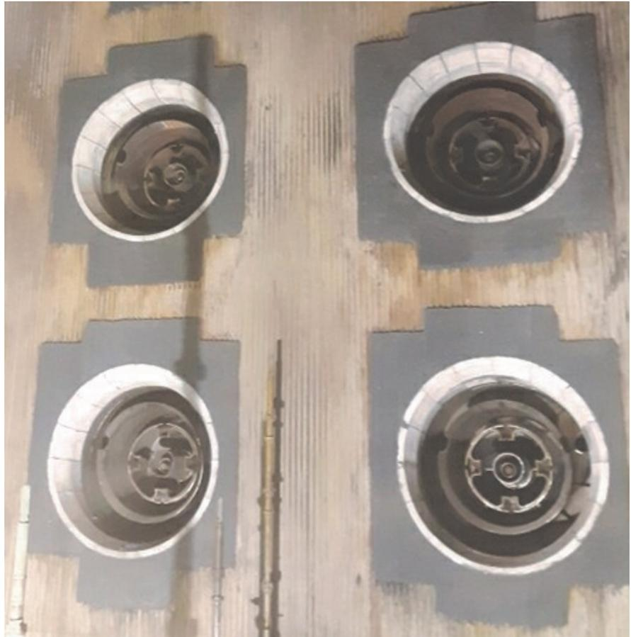
BLACK JACK RAM 80 plastic rammed in the burners of a coal fired boiler.
