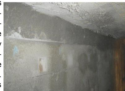
ULTRA TEK 70 NC Wall Cast with top section Shotcreted
